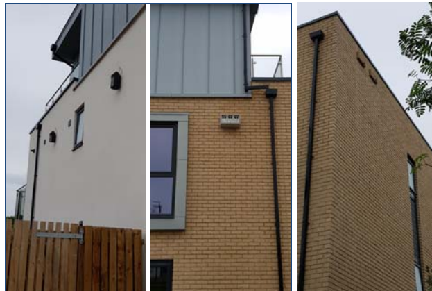
Bat/bird boxes and bricks, Gardener’s Close. Bicester (credit Cherwell Build team)
